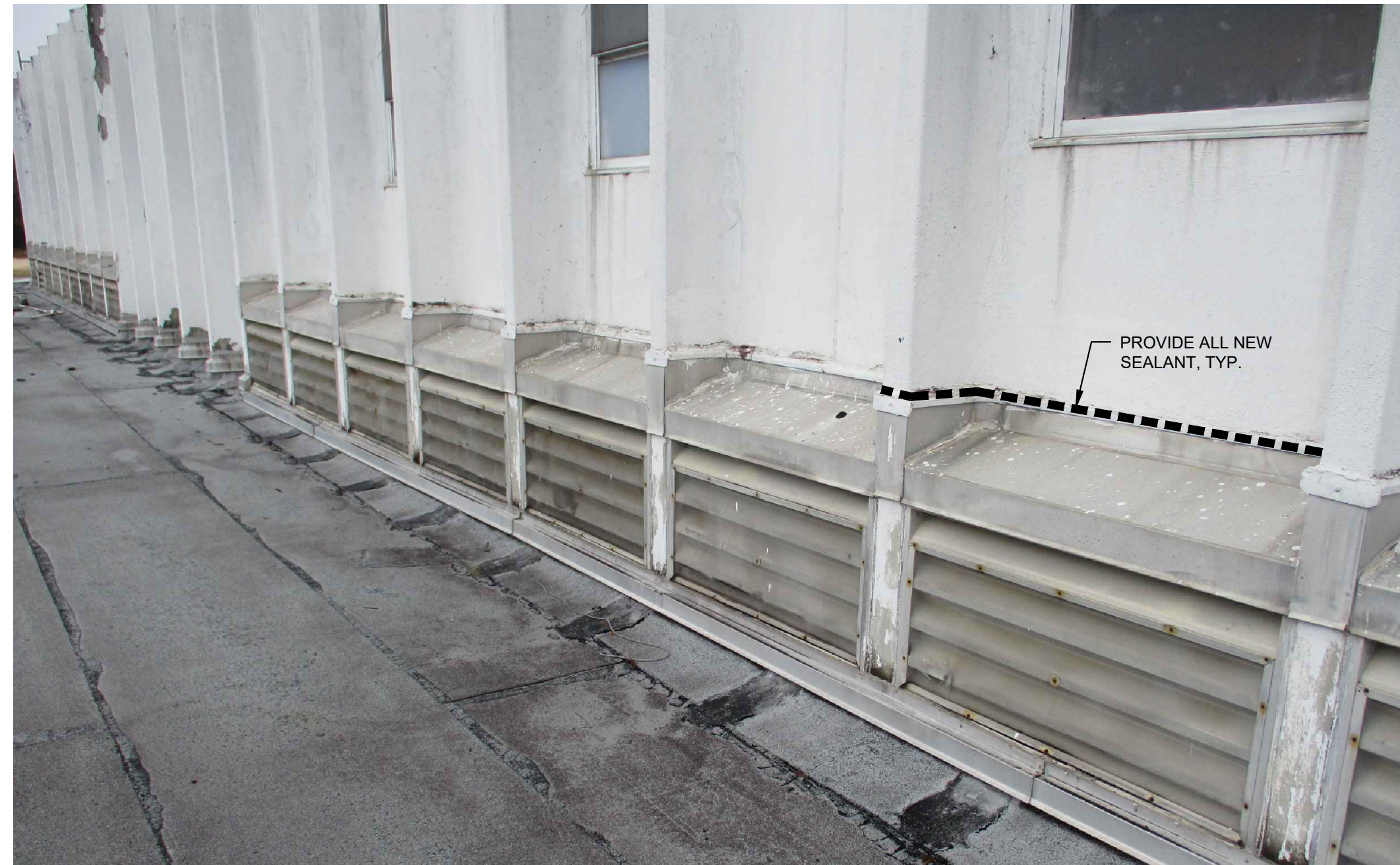
2 SEALANT & FLASHING WORK NOT TO SCALE
